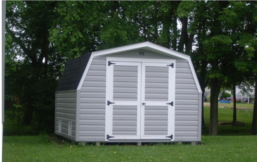
Figure 15: Storage Shed, with Flood Openings (Source: Kevin Wagner, Maryland Department of the Environment)
