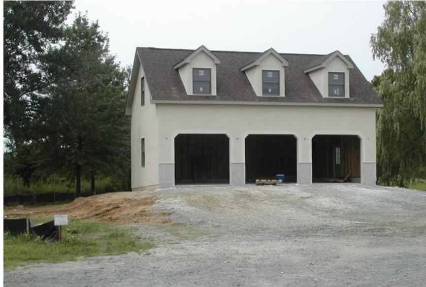
Figure 21: Three-Car Garage Elevated on Fill
