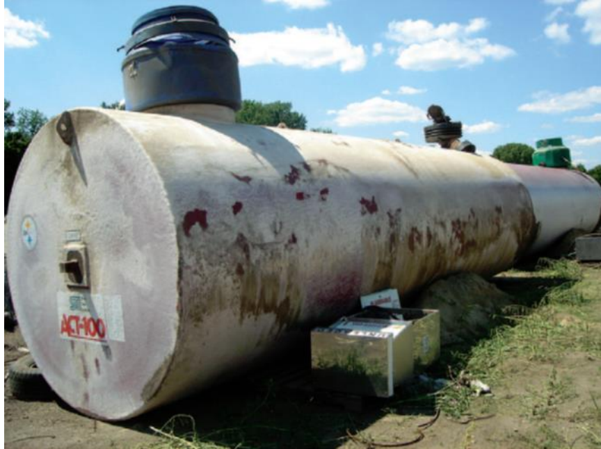
Figure 5: Buoyancy Forces Dislodged Two 10,000-Gallon Underground Fuel Tanks
