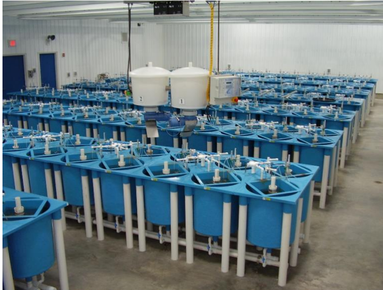
Figure 6: Agricultural Structure Housing Aquaculture Tanks and Equipment (Source: USDA Agricultural Research Service)
