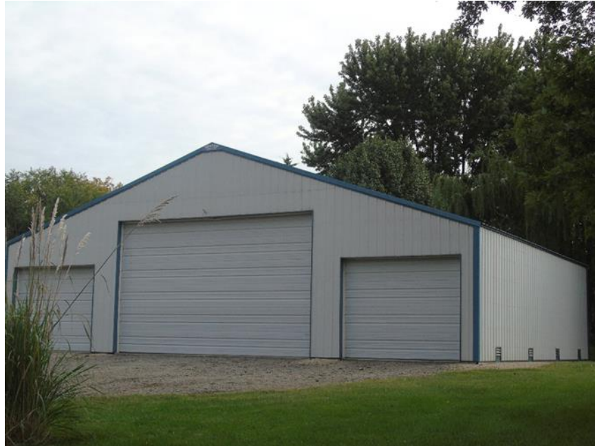
Figure 2: Agricultural Structure for Equipment and Storage, with Flood Openings (Source: Steve Samuelson, Kansas NFIP Coordinator)
