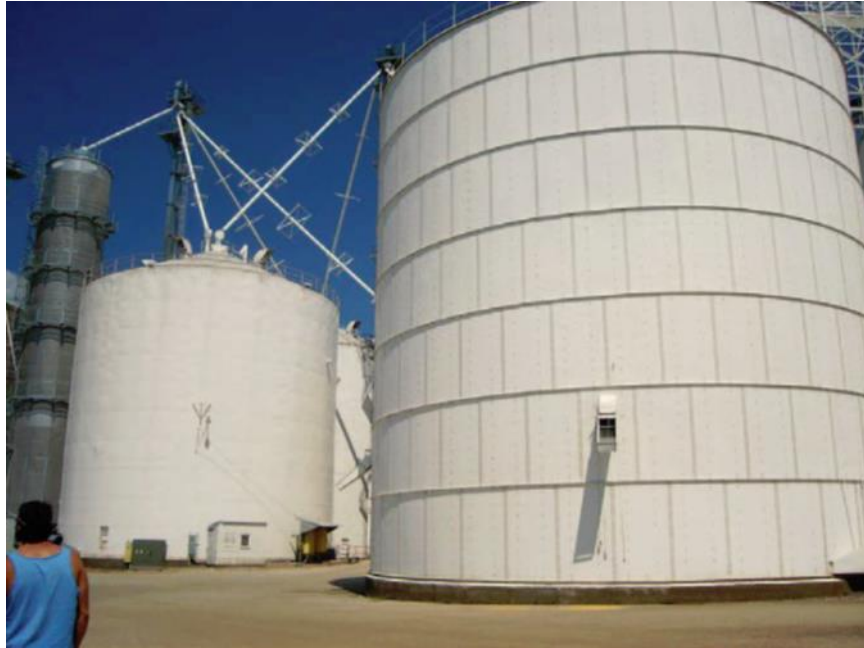
Figure 4: Welded-Seam Silo (Left) May Be Watertight; Bolted-Plate Silo (Right) Is Not Watertight
