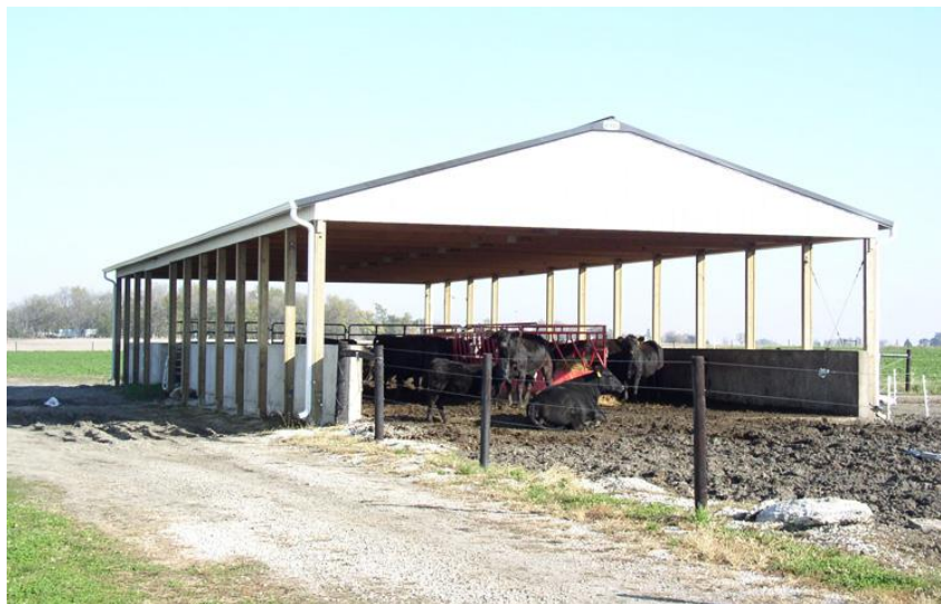
Figure 12: Pole Barn Without Walls (Source: USDA Agricultural Research Service)
