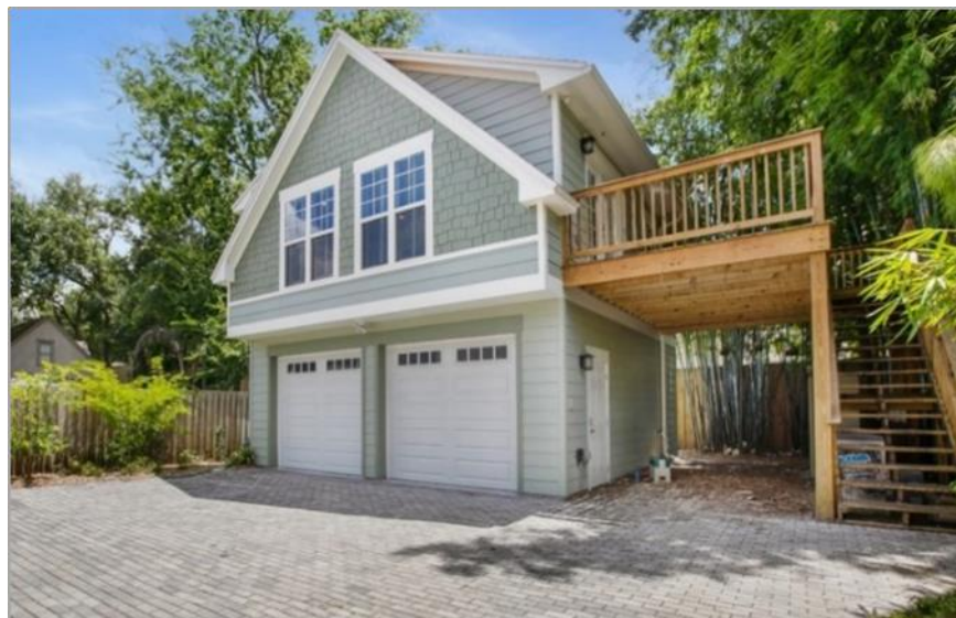
Figure 16: Elevated Accessory Residential Structure, with Enclosure
